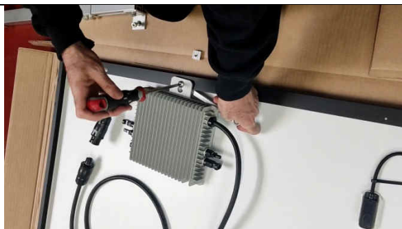
10. On one of the two panels, place the inverter. Use an available hole and screw and tighten the nut to fix the inverter to the panel
